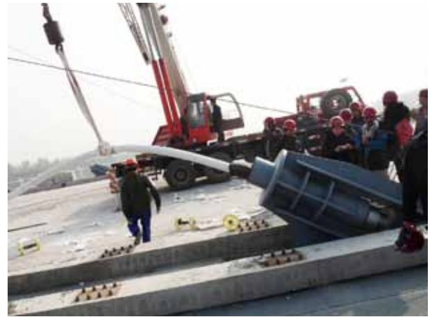
Stay Cable Installation
