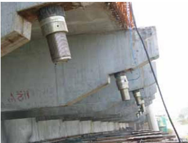
Completed Stay Cables
