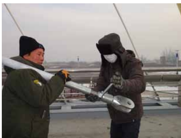
Stay Cable Installation
