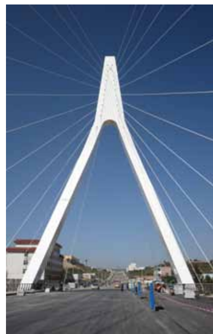
Cable Stayed Bridge
