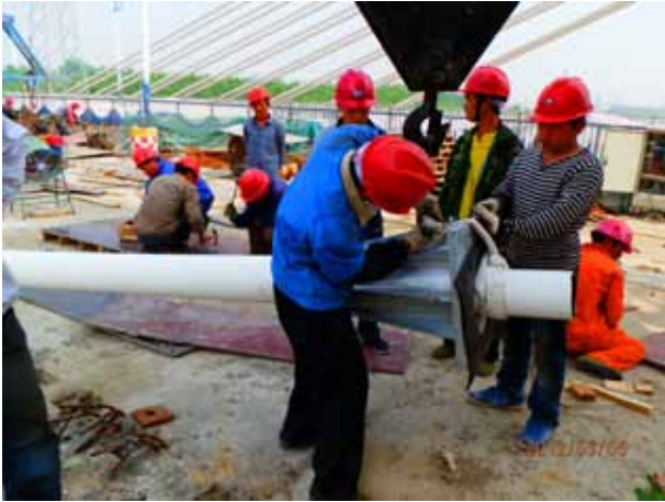
Stay Cable Installation
