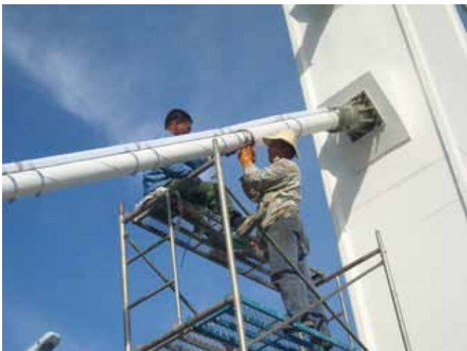
Stay Cable Installation
