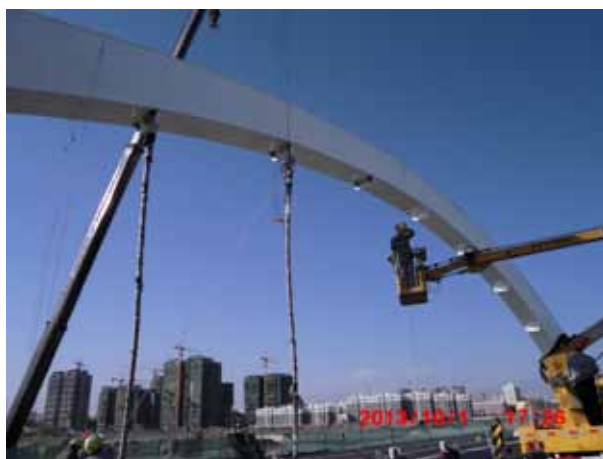
Stay Cable Installation
