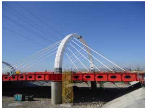
Stay Cable Installation
