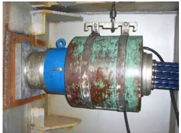
Stressing In Progress
