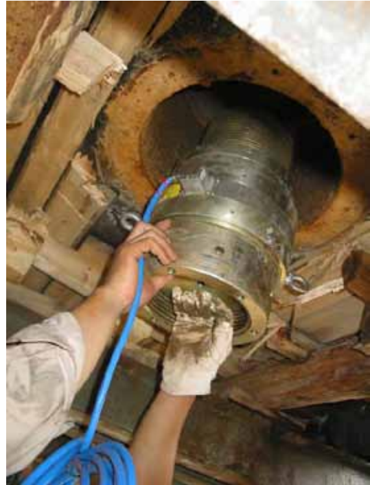
Stay Cable Installation
