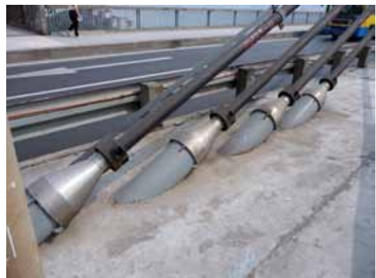
Installed Stay Cables with Waterproof Protection
