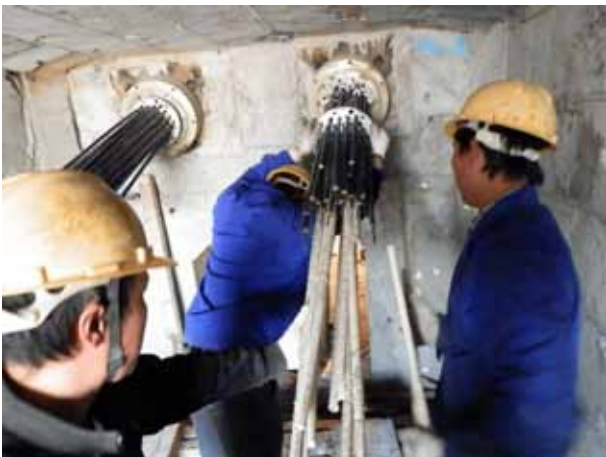
Stay Cable Installation
