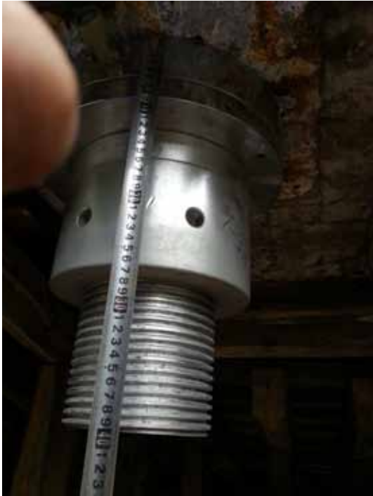
Checking Elongation After Stressing
