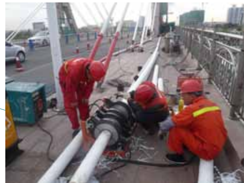
Stay Cable Installation
