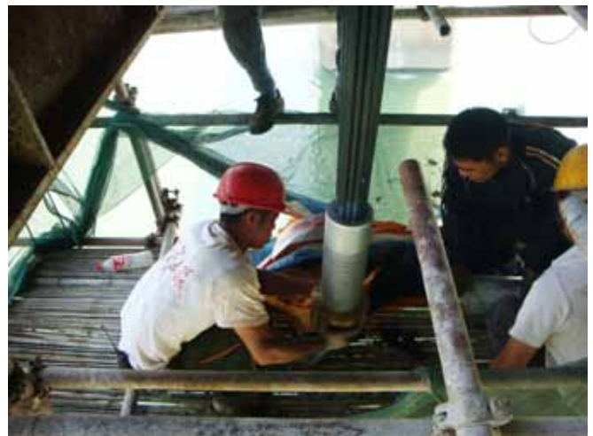
Stay Cable Installation
