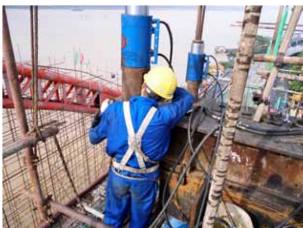
Stay Cable Installation
