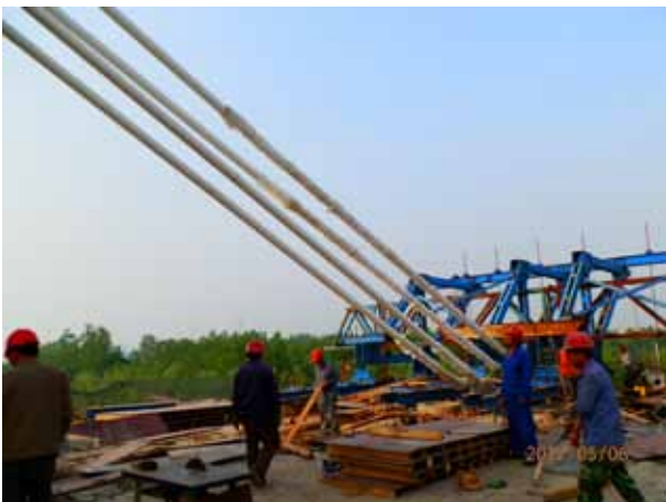
Stay Cable Installation
